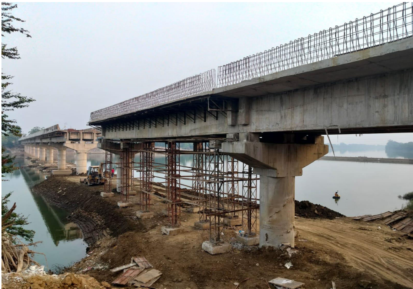
Const. of H.L. Bridge i/c approaches across Shivanarh River on Durg -Nagpura –Karela
