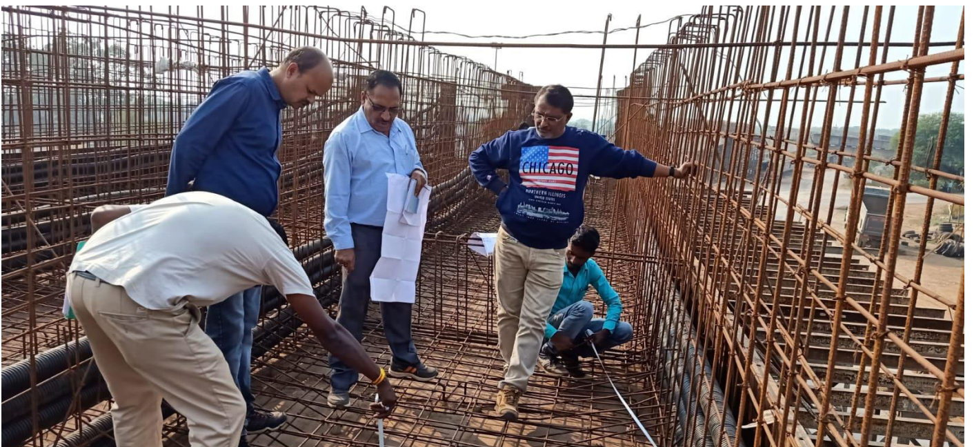
Farhad Chowk Overpass Rajnandgaon –Nagpur Road
