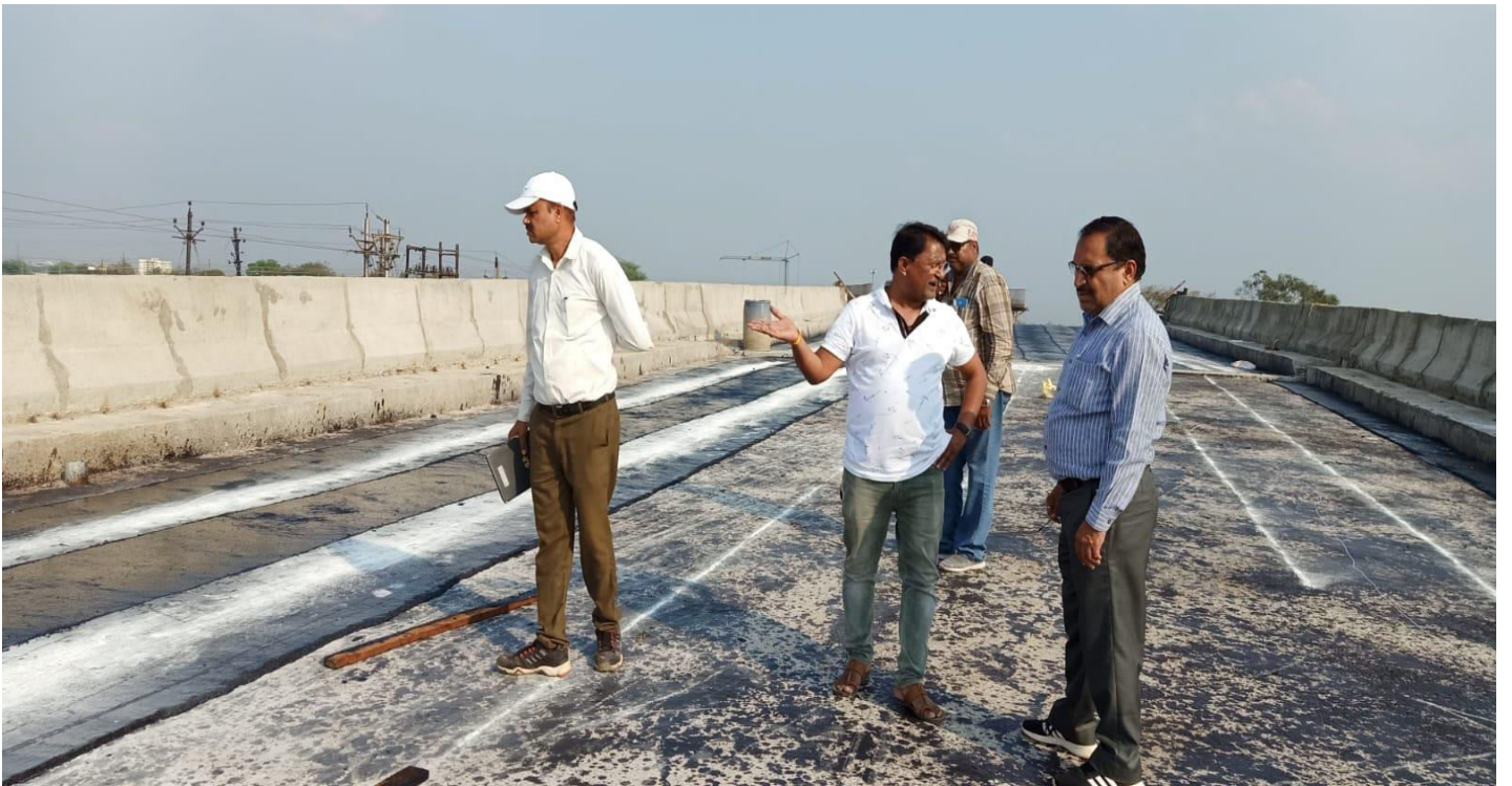
Farhad Chowk Overpass Rajnandgaon –Nagpur Road
