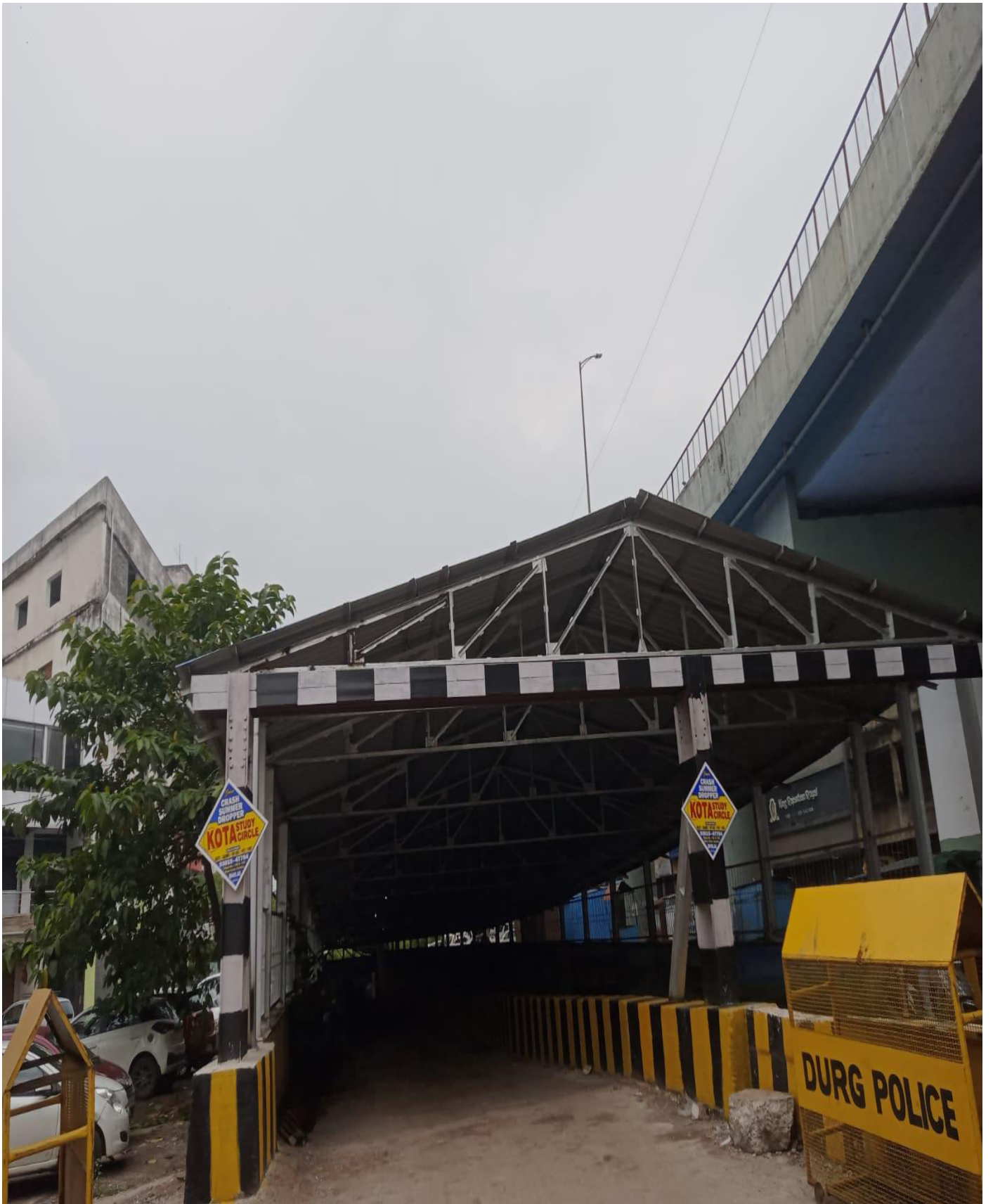
Nehru Nagar Rail Line Under Bridge Bhilai.
